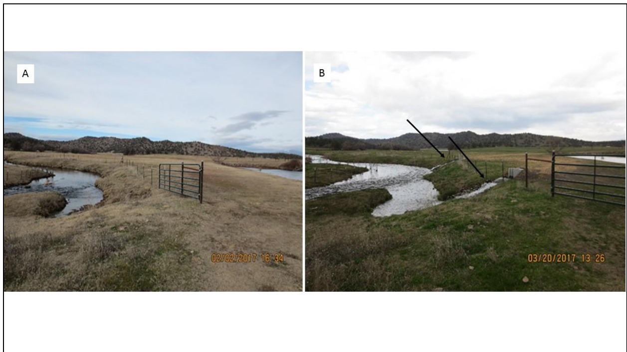
FIGURE 6. PHOTO A) 2017 PRE-PROJECT PHOTO OF NORTH AND SOUTH 105SRHV SPRING PIPELINE SITE; PHOTO B) 2017 POST-PROJECT PHOTO OF NORTH AND SOUTH 105SRHV SPRING PIPELINE OUTLETS (SEE BLACK ARROWS) DISCHARGING COLD (~14°C) SPRING WATER INTO THE SHASTA RIVER.
