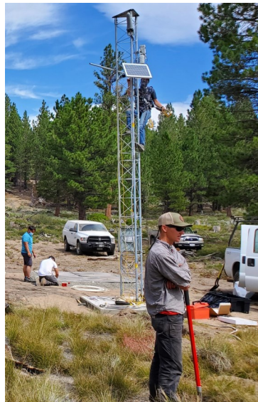
HyDAS Station Construction at Bolam
