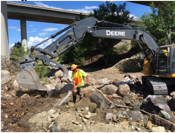
North Rivers Construction placing boulders with Hwy 15 in the background
