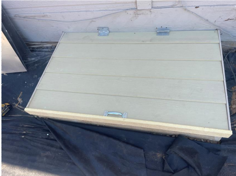
New Crawl Space and Electrical Panel Door built from non-combustible Hardie Board
