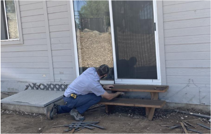
Removing the Combustible Skirting
